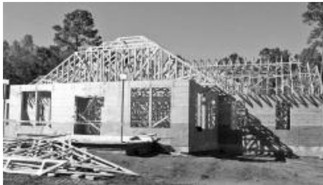
Raising the roof.
